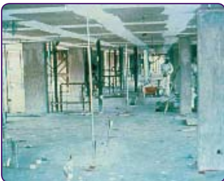
Removal of drywall joint compound now type 2 work.
