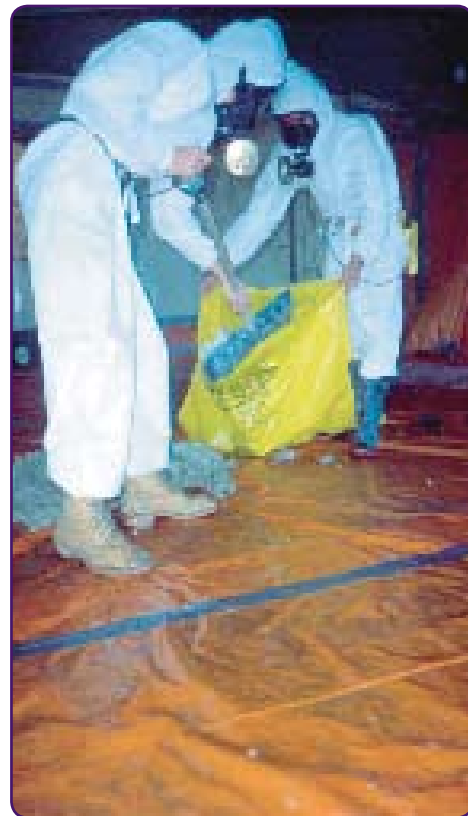
Type 3 removal half face respirators are no longer allowed for type 3 procedures
